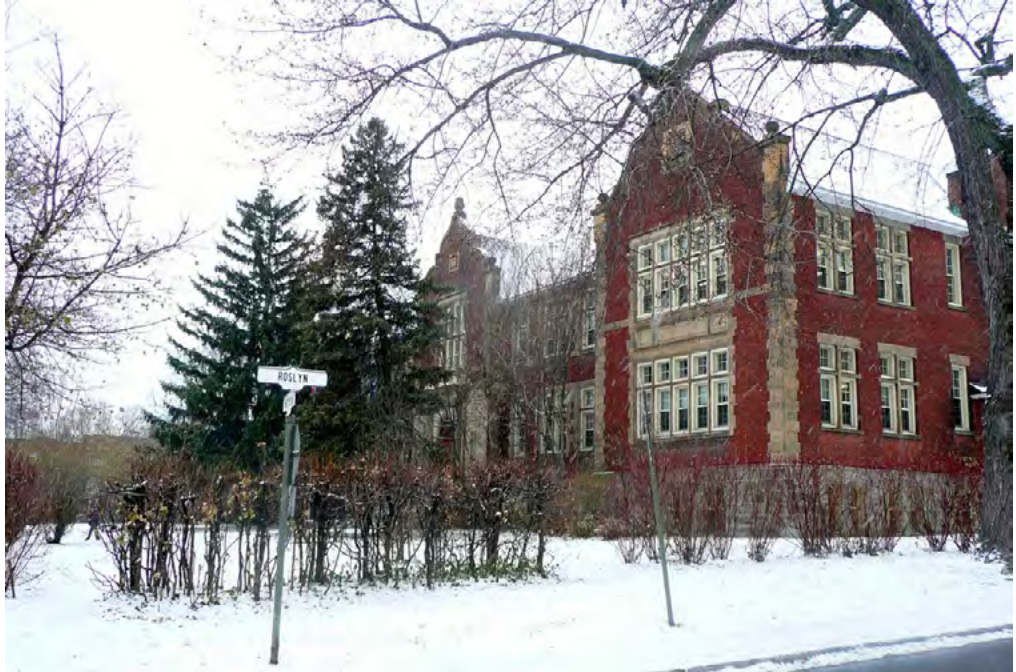
Roslyn Primary School in the Montreal neighborhood of Westmount.
